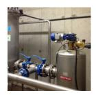
**Well-water**, **geothermal heating**. These filters provide an efficient solution for well-water filtration (geothermal heating, irrigation, etc.), even in the presence of clay or fine mud.
